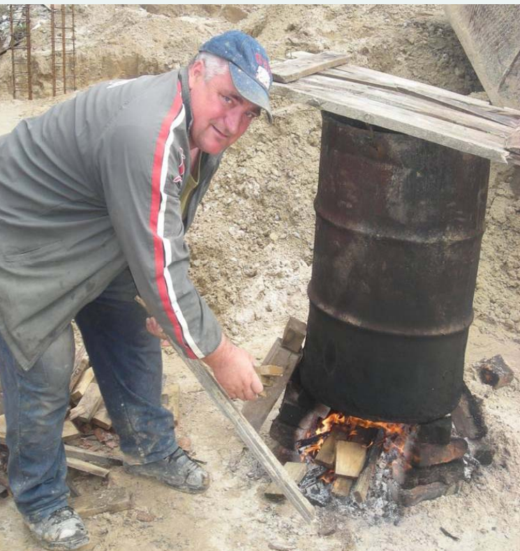
Vyacheslav lights a fire to heat the pitch to seal the crypt church's outer walls from destructive moisture in Lutsk
