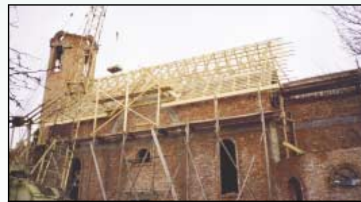
Church construction in Khust.
