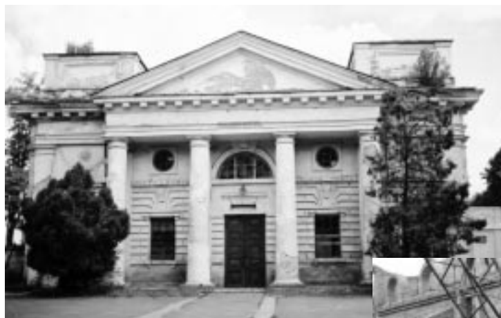
Assumption of Virgin Mary church in Smila needs many repairs.
