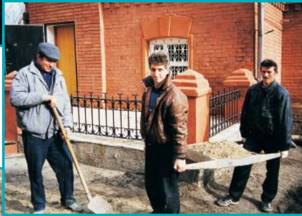
Church Repair in Penza.
